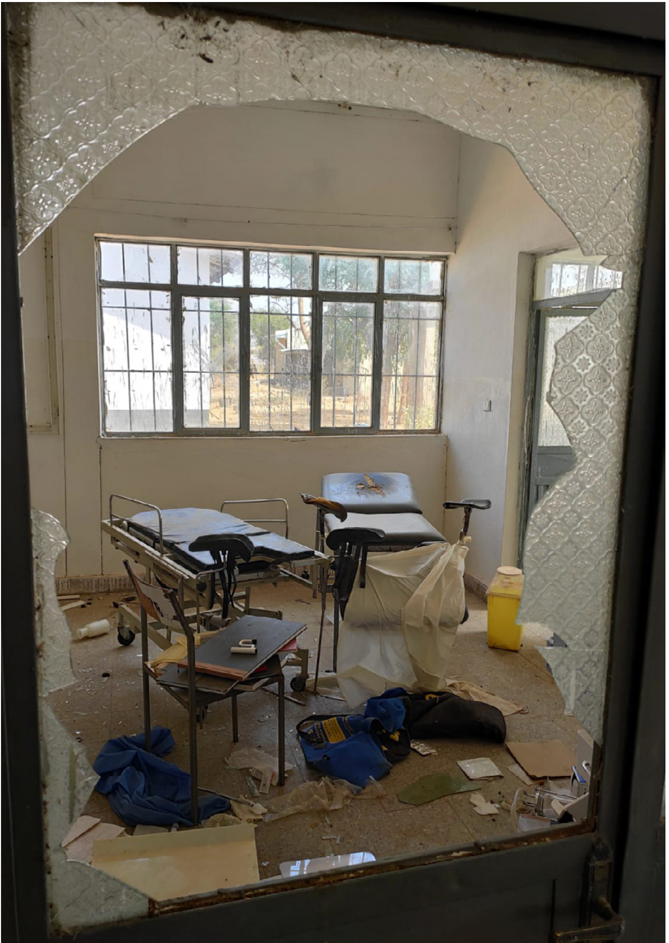
↑ Damaged OT room in Sheraro hospital. Ethiopia, March 2021. Photo: MSF.
